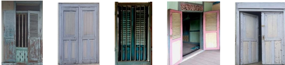
Figure 13. sample house door and window shapes (wooden slatted windows and wooden doors)
