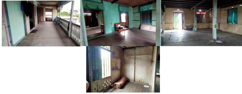
Figure 12. Photo of the existing interior space in the sample building
