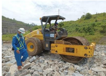
Figure 14. Rockfill Compaction Using 12 Ton Vibro Roller
