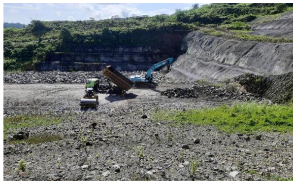
Figure 12. Dumping Material Rockfill Quarry
